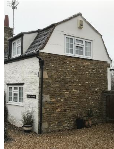
Example of mansard roof
